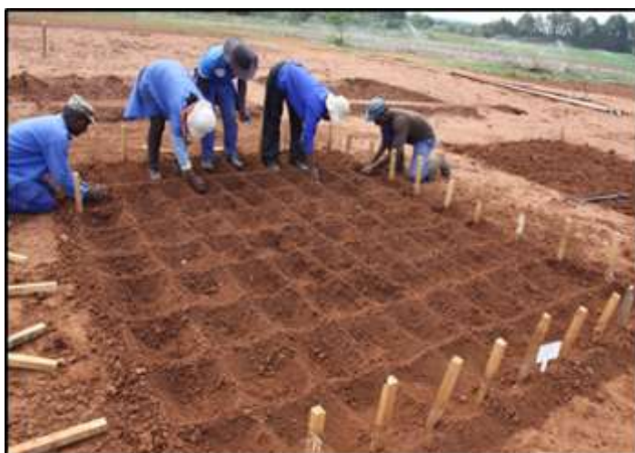
Figure 6. Construction of the in-situ rainwater harvesting and conservation planting pits at Roodeplaat, ARC-VIMP.
