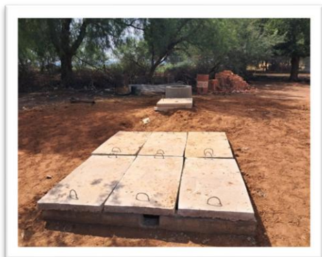
Complete biogas digester connected to the gas stove
