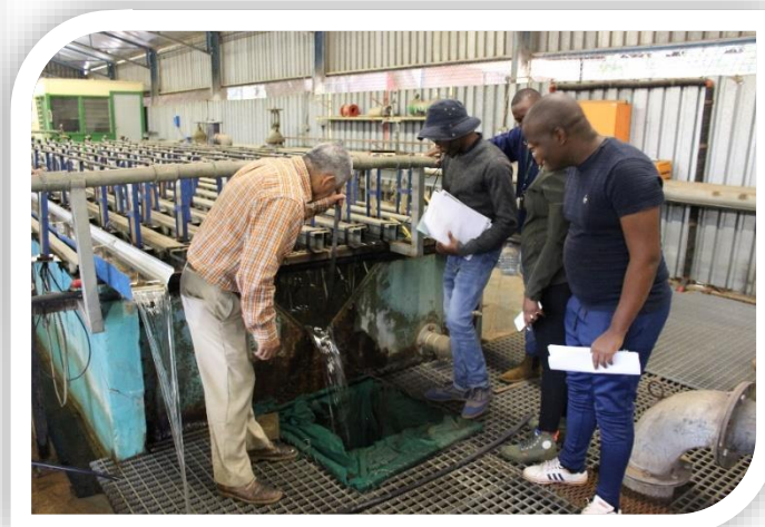
Mr Petersen explaining the water flow through a V-notch weir
