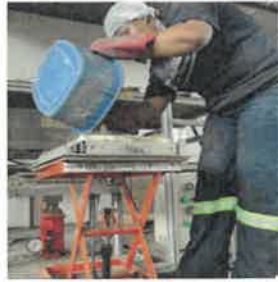
Loading the mixture into the form
