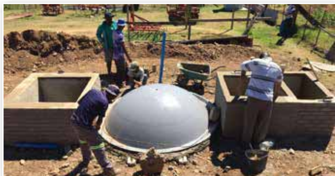
Construction of a bio-digester in Krwakwa village, Eastern Cape.
