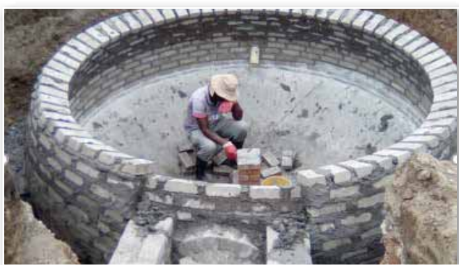
12 m 3 brick biogas digester.
