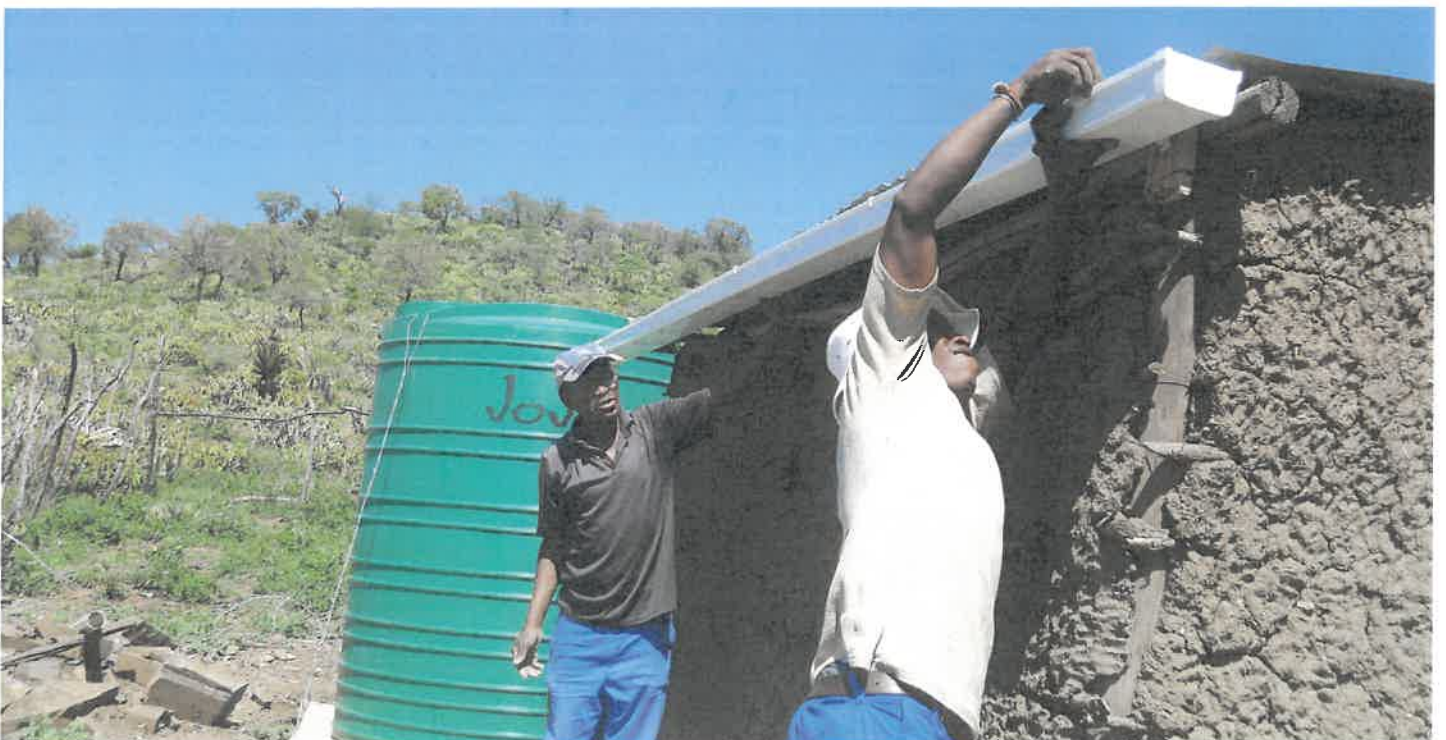
Figure 5. Fitting of gutters to a roof to allow collection of rainwater
