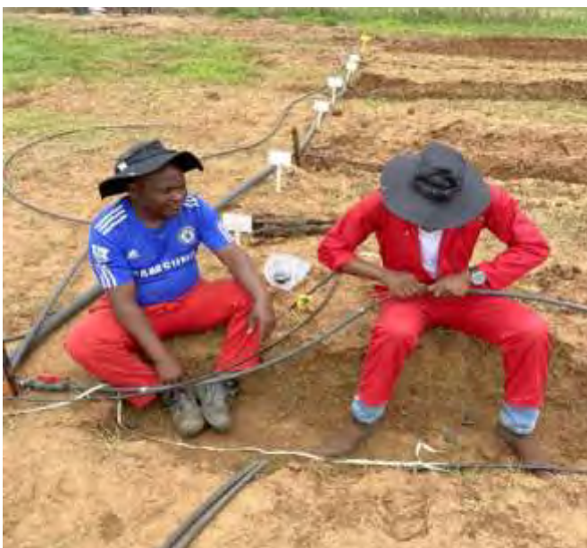
Figure 1. Subsurface drip irrigation system installation underway at the ARC.
